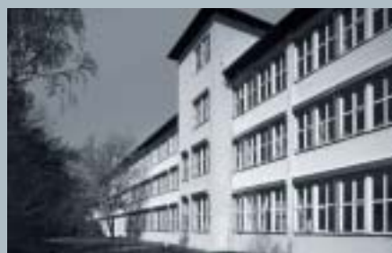
Left: Our location in St. Georgen Right: Our location in Landshut
